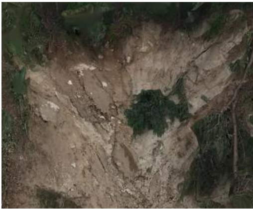
(c) Close-up photo of the collapse site
