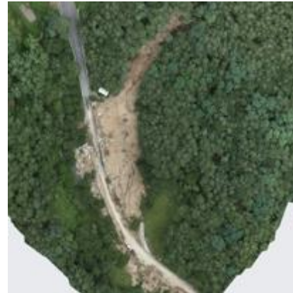
(b) Overall view 2
