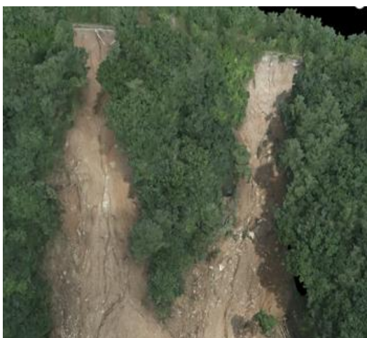
(b) Close-up photo of the collapse site
