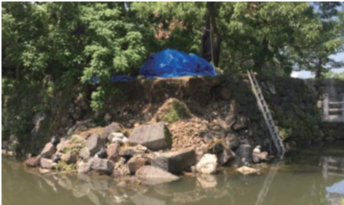
Figure 3: condition of the collapsed stone wall at the bridge gate
