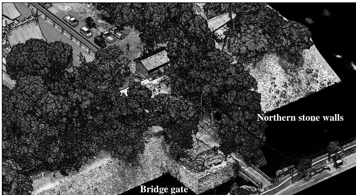
Figure 6: Example of Acquired Data (Bridge gate and Main tower foundation)
