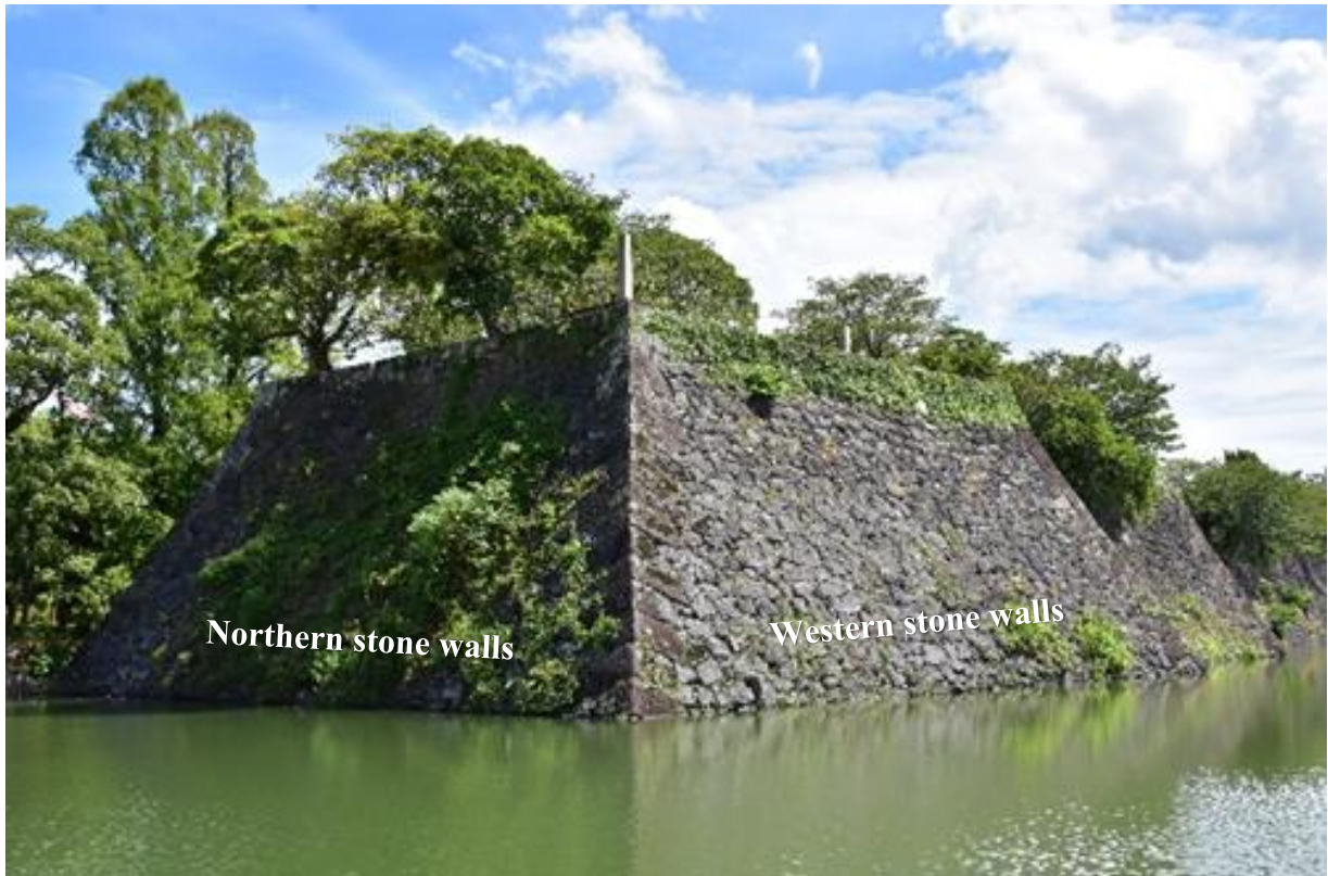
Figure 4: Stone walls at the Main tower foundation
