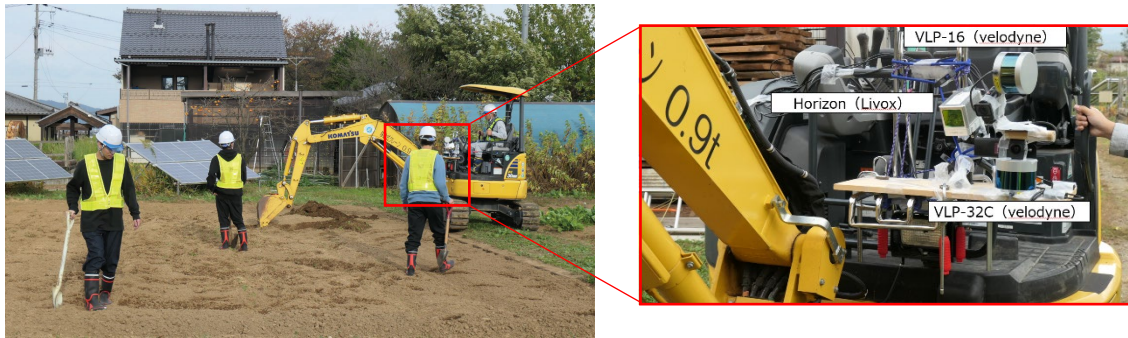
Figure 8: Simulated construction space and mounted LiDARs.
