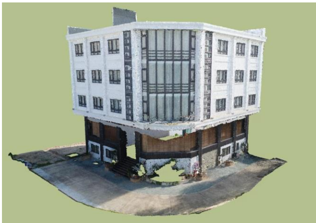
Figure 4: Point cloud of a detached house which is built from UAV images
